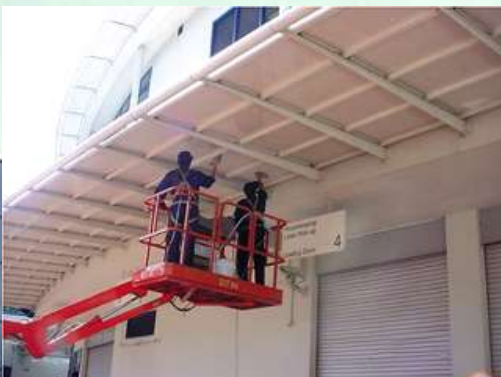
Cleaning of podium block using mobile boom lift
