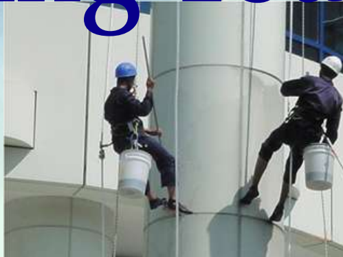
Cleaning of pillars using robe access
